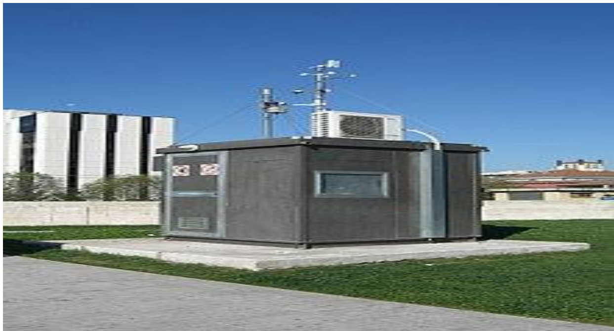
Figure2: Air quality monitoring station
